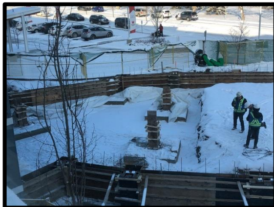
Second concrete footing pour for the new Chapel
